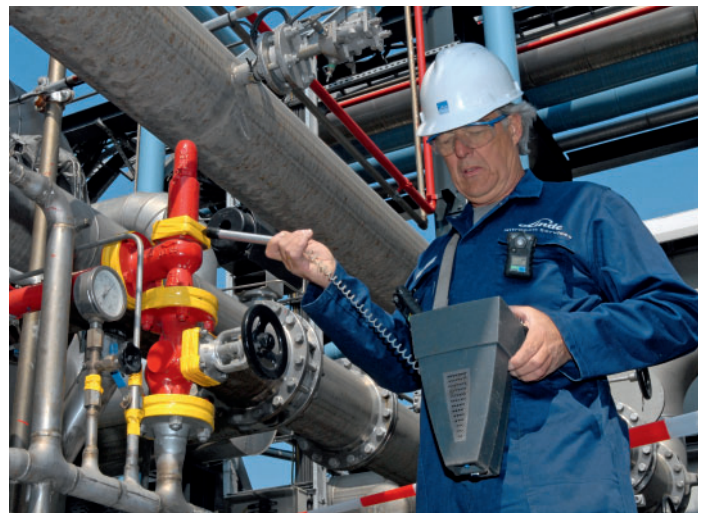
Application of a nitrogen/helium mixture for leak testing
